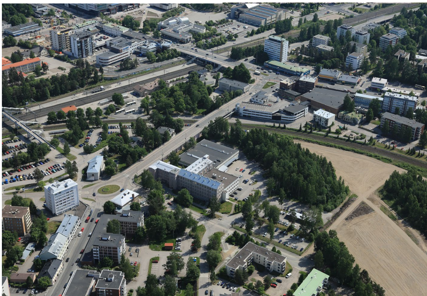
Aerial view from southwest
